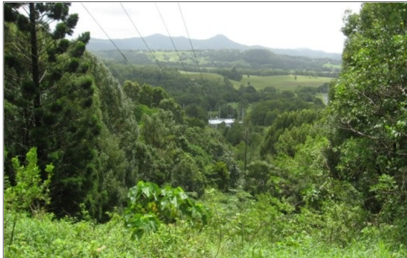
The view from pipehead down to the power station Photo - Gary Estcourt.
