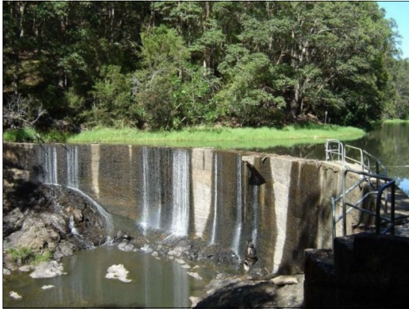
The Mullumbimby Hydro-electric Scheme weir on Wilson's Creek.
