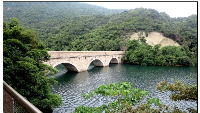
One of 4 masonry bridges along the western shore of the reservoir, bridging major inflowing streams.
