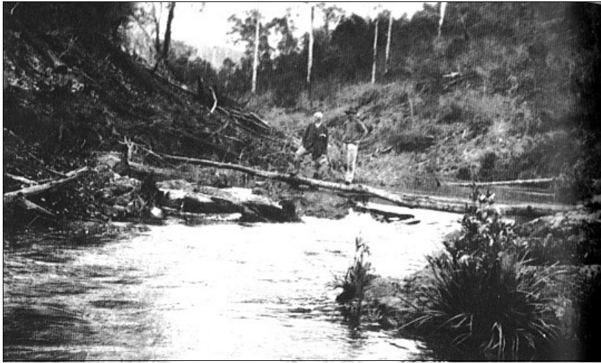
Examining the site for the future Power Station weir in 1924 - from Brokenshire p.76. Could the gentleman on the left be design Engineer William Corin?
