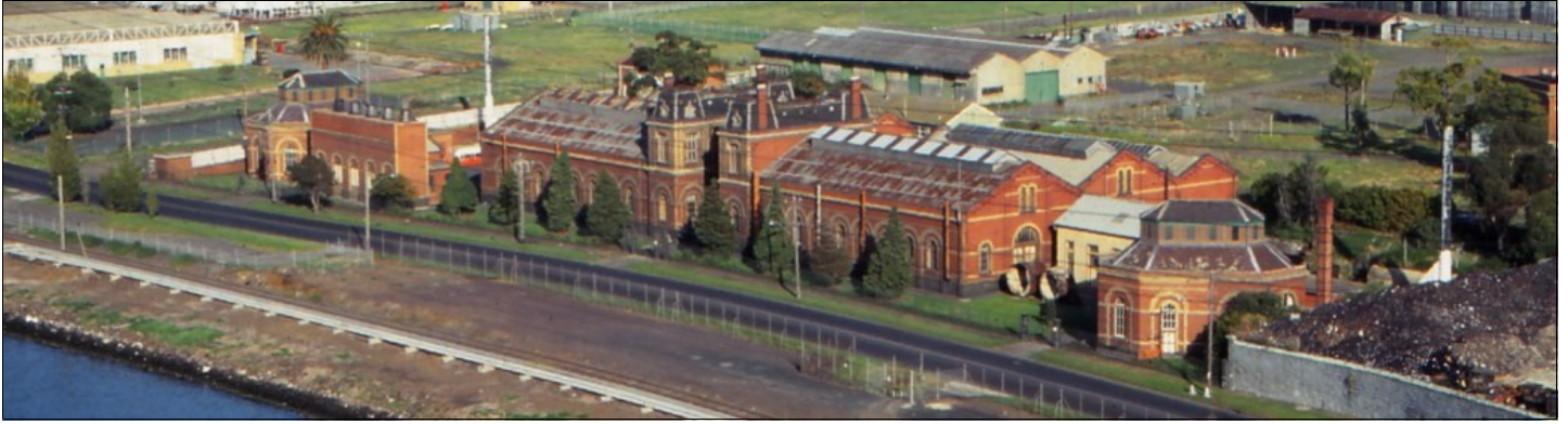
Spotswood Sewage Pumping Station viewed from the Westgate Bridge in May 1985
