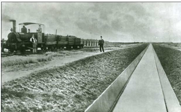
Building the Main Outfall Sewer Aqueduct. Image - Culture Victoria.
