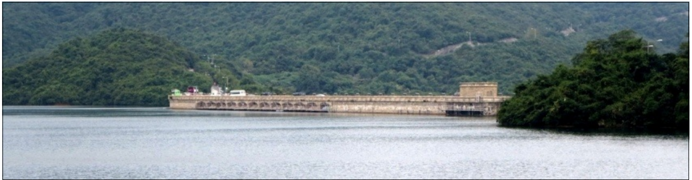
The Tai Tam Tuk Reservoir Dam, with the Tai Tam Road passing over its 12 spillways
