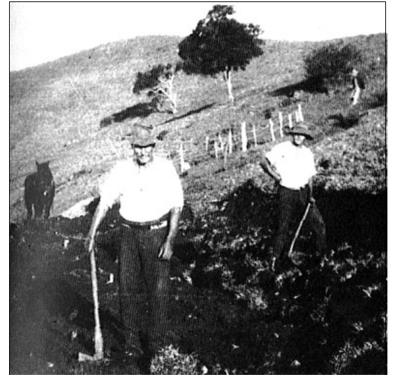
Another image from Jim Brokenshire's book, showing Mr Davidson, ex-Mayor of Mullumbimby and an original supporter of the hydro scheme, at work excavating for the pipehead reservoir.
